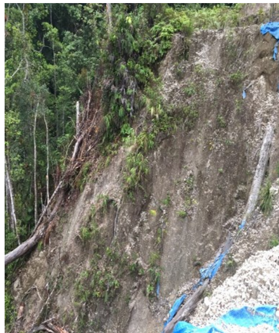
Figure 2. Landslide caused by road construction at Karai watershed.
